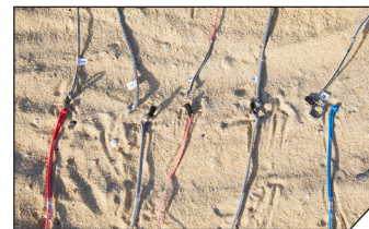
14 Connect flying lines to the pigtails using the number label system.
